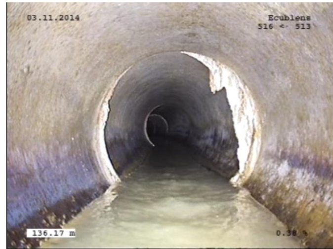
Calcaire aux joints
