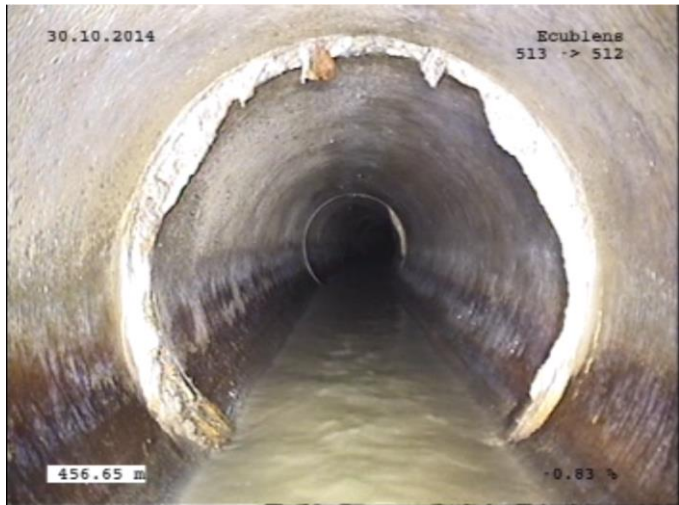
Calcaire aux joints
