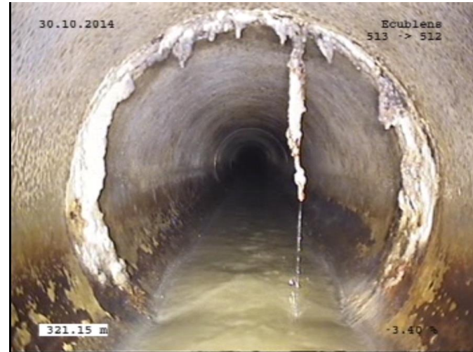
Calcaire aux joints
