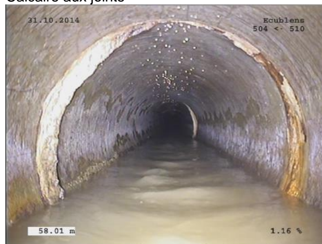
Calcaire aux joints
