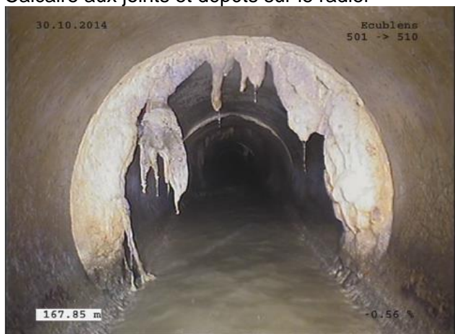
Calcaire aux joints
