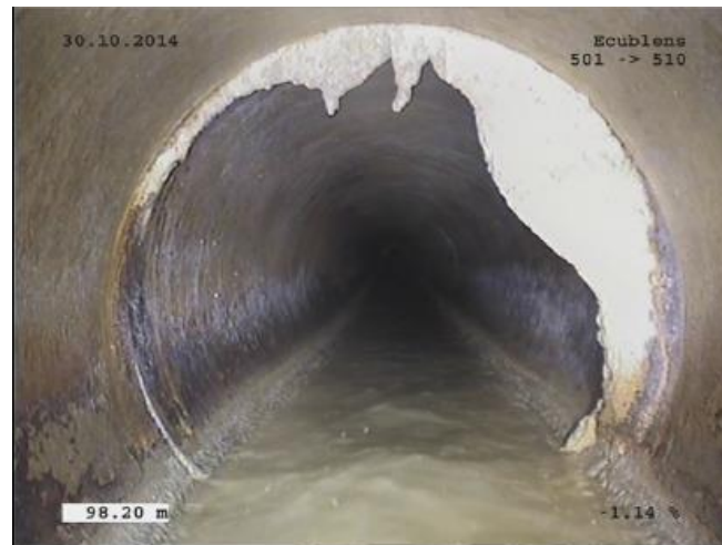
Calcaire aux joints
